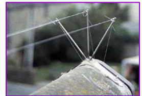
Horizontal sprung wires for Skilled installation above ledges, pipes, signs etc
